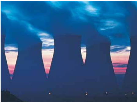
Power Generation Plants
